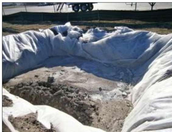
Plate 5-13 Concrete Washout Area
